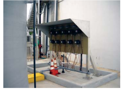
Photo 2. Permanent pumping system for supplemental carbon.
