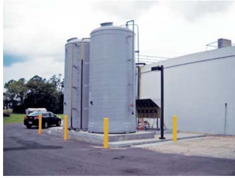
Photo 1. Permanent supplemental carbon bulk storage and pumping system at the Westside Regional Water Reclamation Facility in Daytona Beach.
