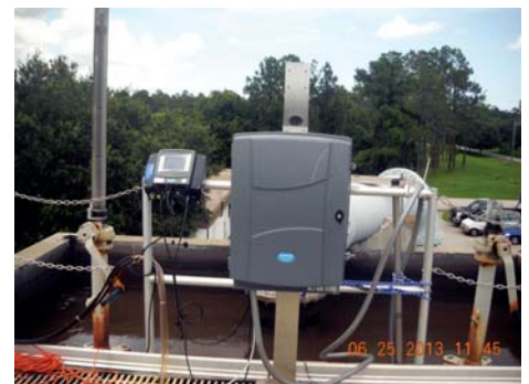
Photo 4. Orthophosphate on-line analyzer located in the influent to the anaerobic zone at the Westside Regional Water Reclamation Facility to record real-time influent phosphorus loading during the study.
