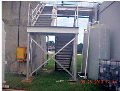
Photo 3. Temporary bulk storage and feed/pumping system used for supplemental carbon at the Westside Regional Water Reclamation Facility during the study.
